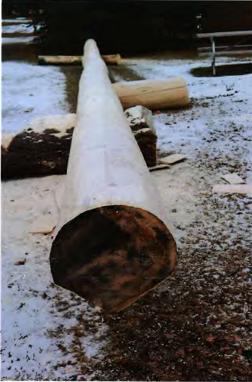
Center roof support beam – dressed.
