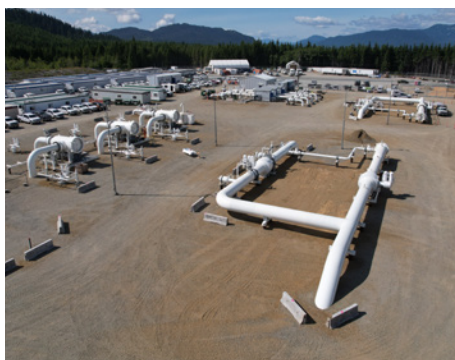
The Kitimat Meter Station, where natural gas will be inspected, measured and then delivered to the LNG Canada facility.
