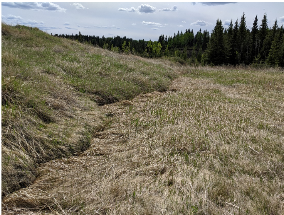
Photo 9 - Crack in soil observed at toe of slope along west side of landfill. Looking south.
