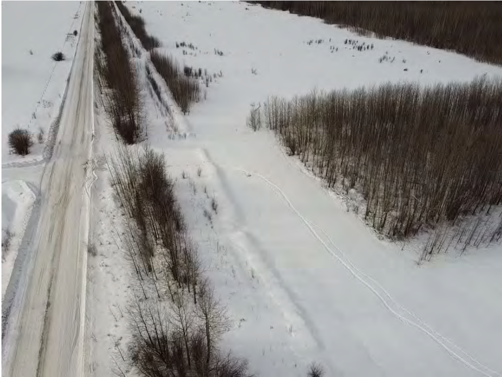
Overview of existing approach at crossing 1 and 2.
