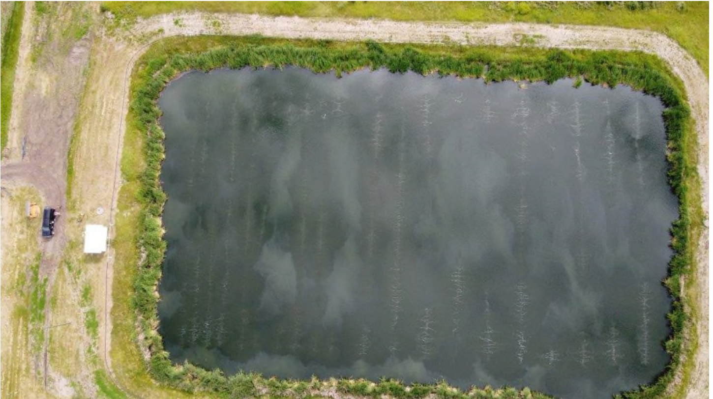
Figure 7: Aeration Lagoon Aerial Photo from Assessment Site Visit (2020-07-28)
