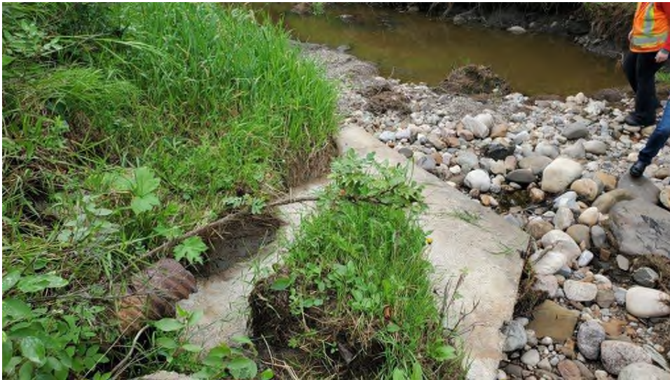
Figure 13: Outfall Structure Photo from Assessment Site Visit (2020-07-28)
