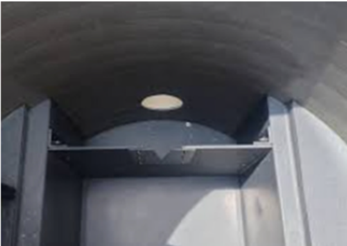
Figure 14 - Example of V-Notch Weir
