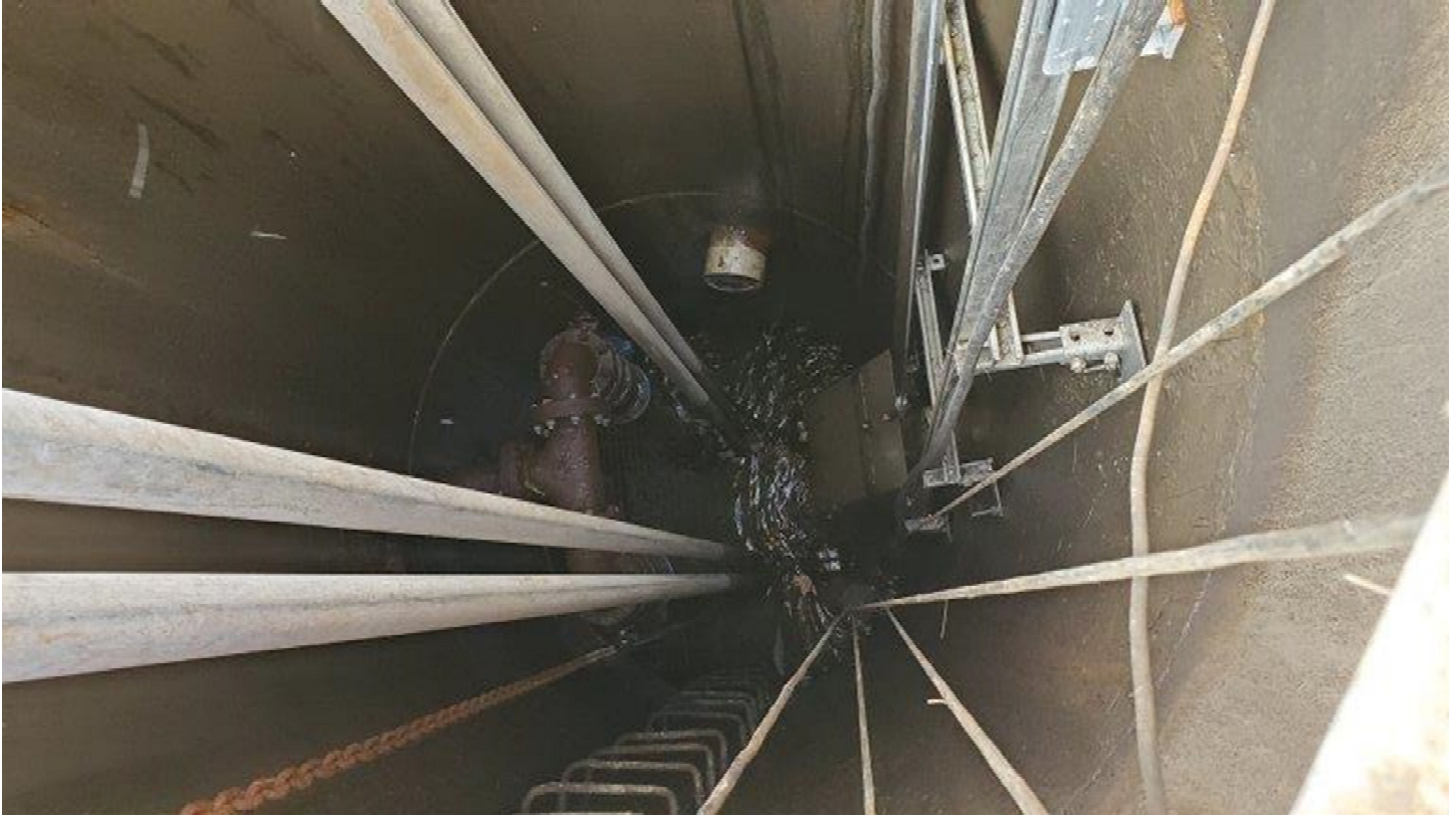
Figure 5: Lift Station Manhole Photo from Assessment Site Visit (2020-07-28)
