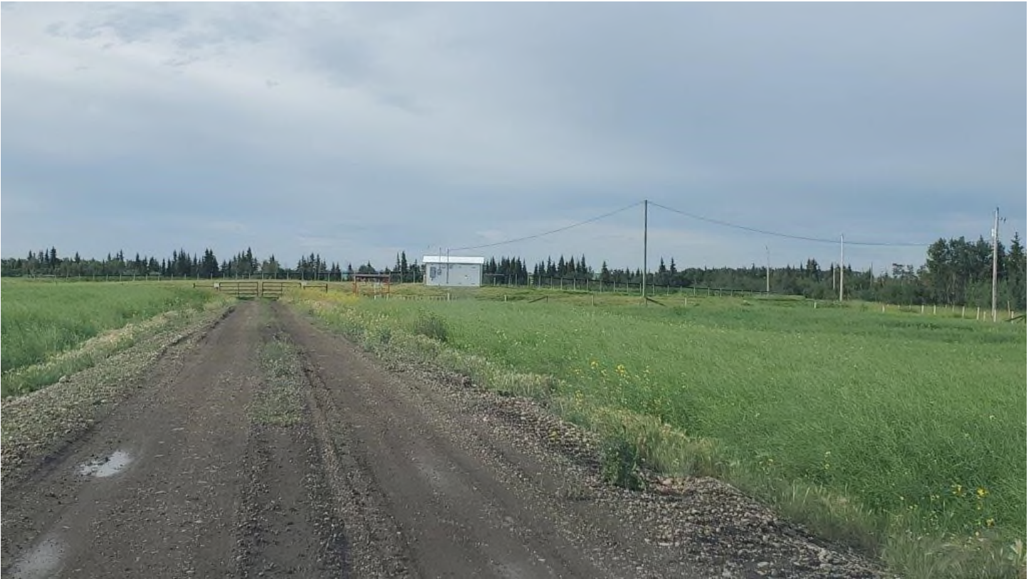
Figure 3: Access Road Photo from Assessment Site Visit (2020-07-28)
