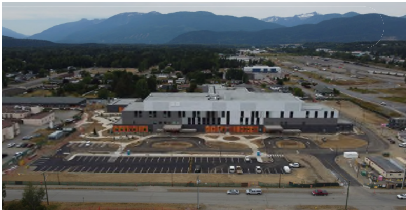
Landscaping & Civil (East Side)
