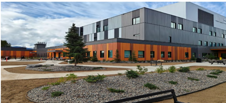
Landscaping & Civil (East Side)
