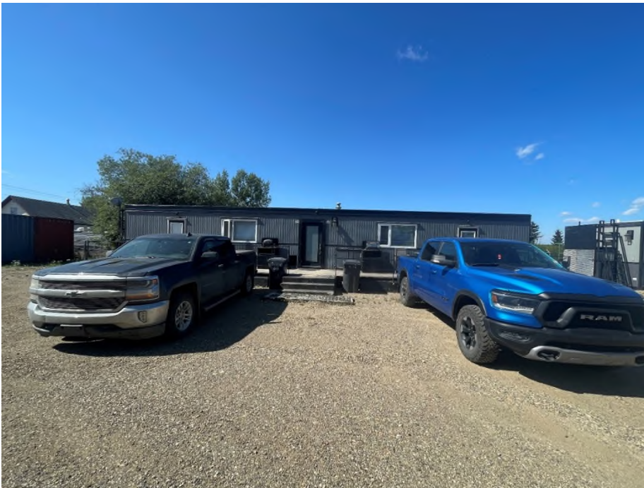
Photo of the southernmost dwelling structure on the Property
