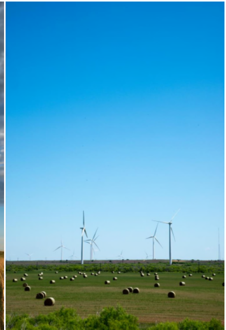
Taylor Wind - EDF Renewables Canada Inc | 15
