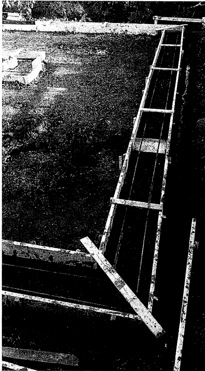
Figure 1. Footing installed on stable native soil. Continuous 15M rebar installed
