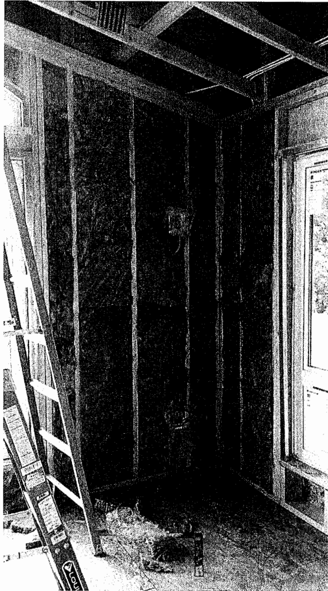
Figure 7. 5.5" batt insulation inside 2x6 walls and start of vapour barrier.
