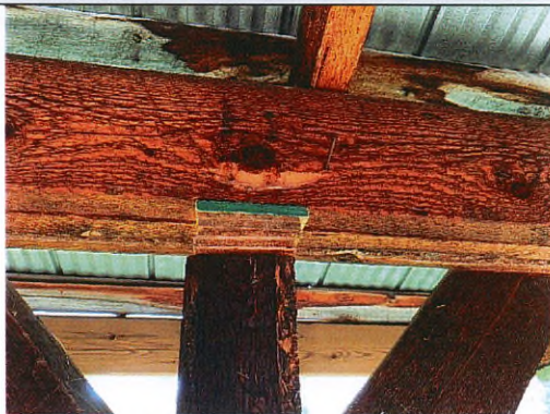
plywood shims column to beam
