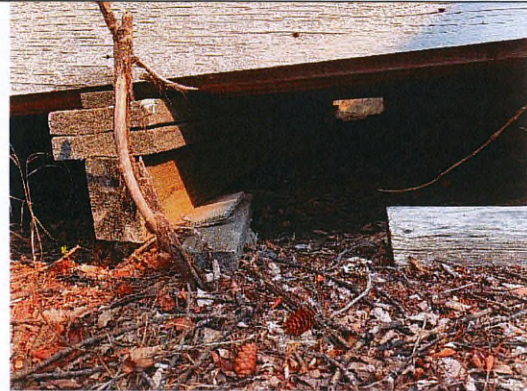
Untreated timber foundation
