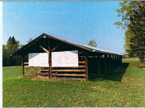
Roof sagging in various locations
