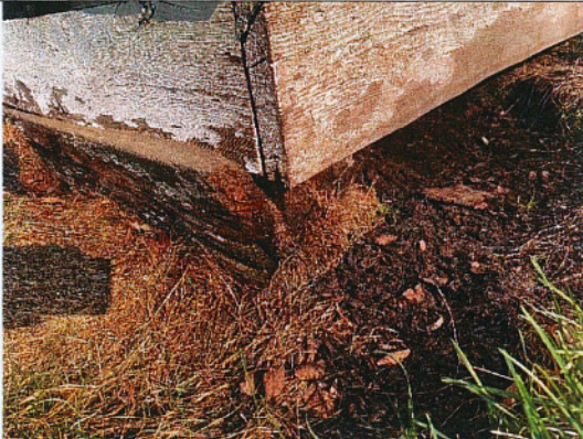
Untreated timber foundation on ground
