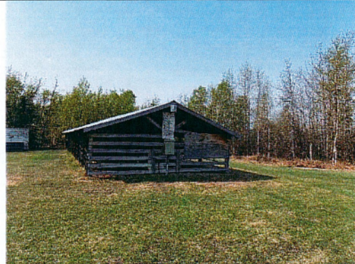
Roof sagging in various locations
