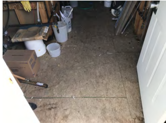
North Peace Fair Grounds - Washroom Building - B101001
