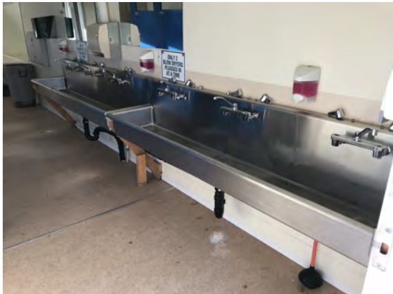
North Peace Fair Grounds - Washroom Building - D201003
