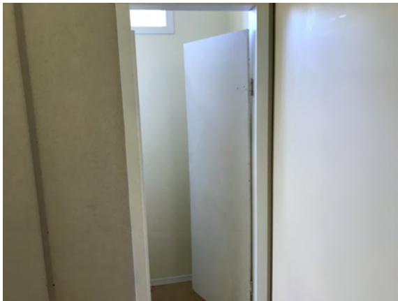
North Peace Fair Grounds - Washroom Building - C301005
