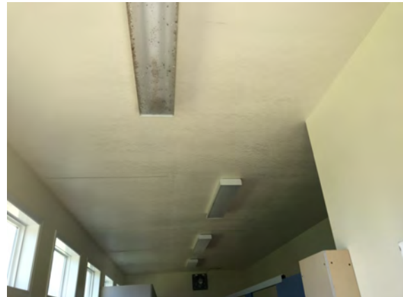
North Peace Fair Grounds - Washroom Building - D502002
