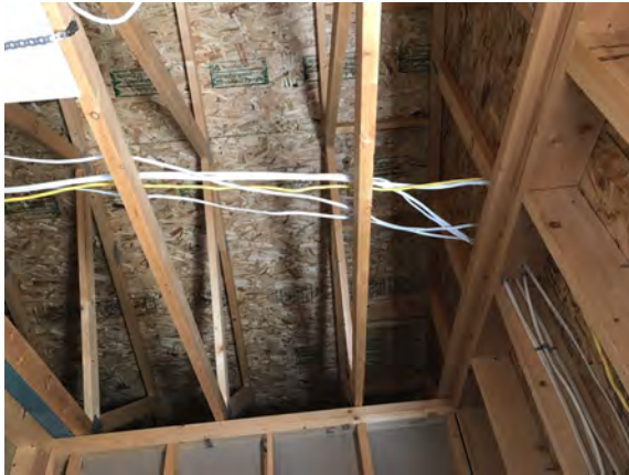
North Peace Fair Grounds - Washroom Building - D502001
