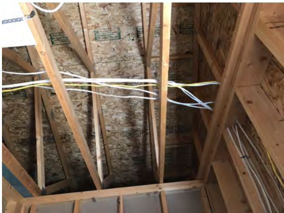
North Peace Fair Grounds - Washroom Building - B103001
