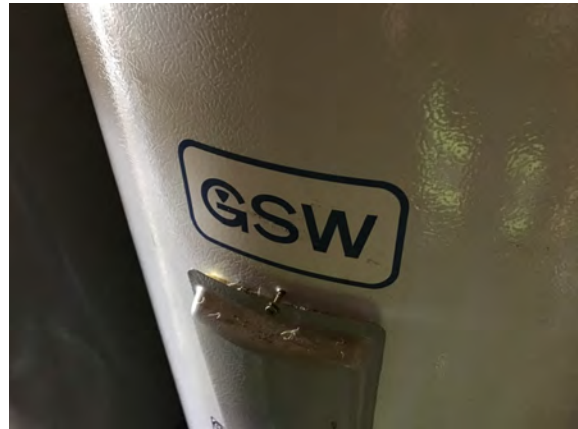
North Peace Fair Grounds - Washroom Building - D202033
