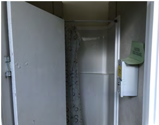
North Peace Fair Grounds - Washroom Building - D201043
