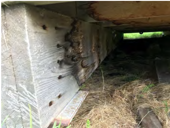
North Peace Fair Grounds - Washroom Building - A101001
