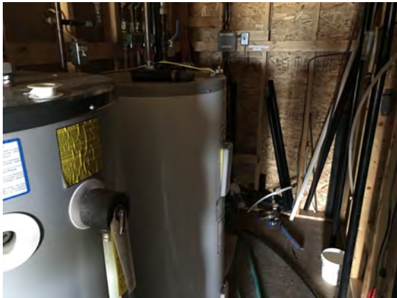
North Peace Fair Grounds - Washroom Building - D202033
