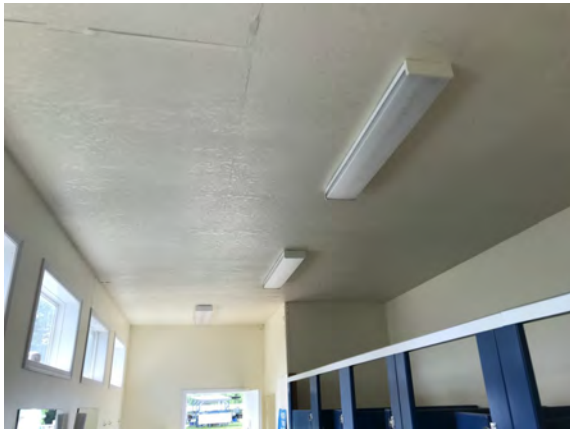
North Peace Fair Grounds - Washroom Building - C303006
