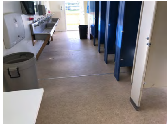
North Peace Fair Grounds - Washroom Building - C302023
