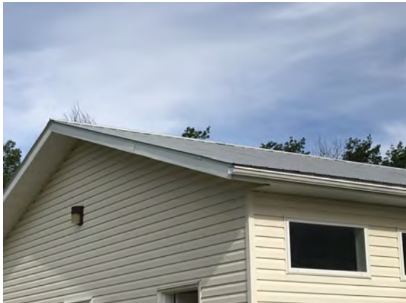
North Peace Fair Grounds - Washroom Building - B301027
