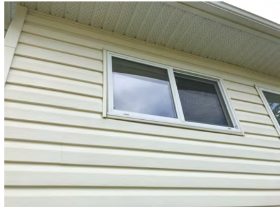
North Peace Fair Grounds - Washroom Building - B202001
