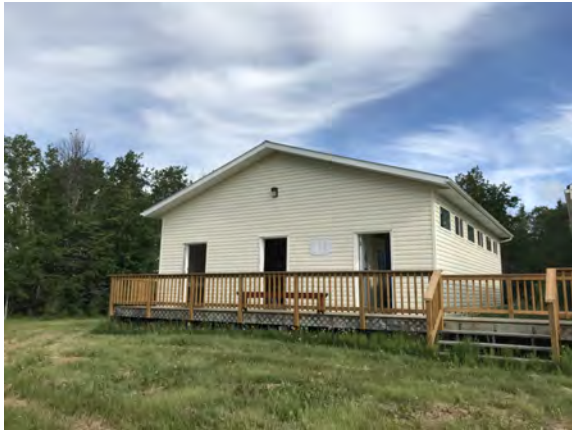
North Peace Fair Grounds - Washroom Building - B201025
