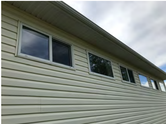
North Peace Fair Grounds - Washroom Building - B202001
