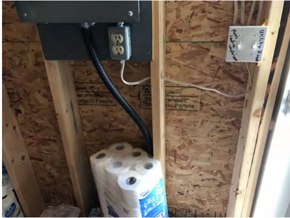
North Peace Fair Grounds - Washroom Building - D502001
