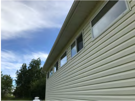
North Peace Fair Grounds - Washroom Building - B201025
