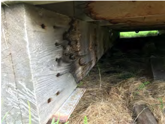
North Peace Fair Grounds - Washroom Building - B101001
