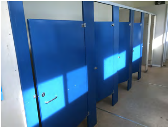
North Peace Fair Grounds - Washroom Building - C103026
