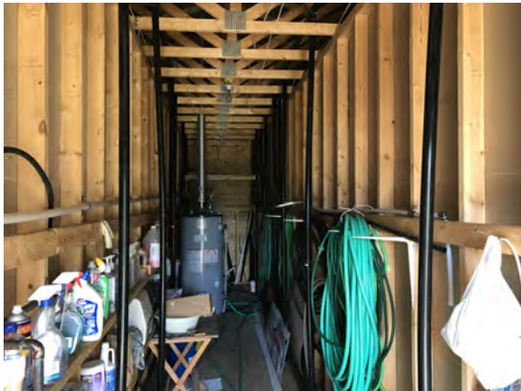
North Peace Fair Grounds - Washroom Building - B103001
