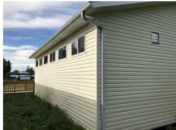
North Peace Fair Grounds - Washroom Building - B301005
