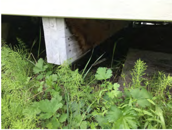
North Peace Fair Grounds - Washroom Building - A101001
