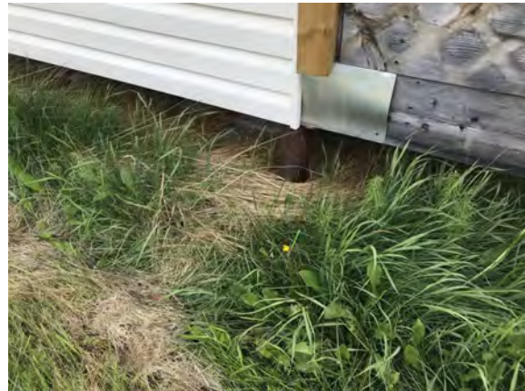
North Peace Fair Grounds - Washroom Building - A101001
