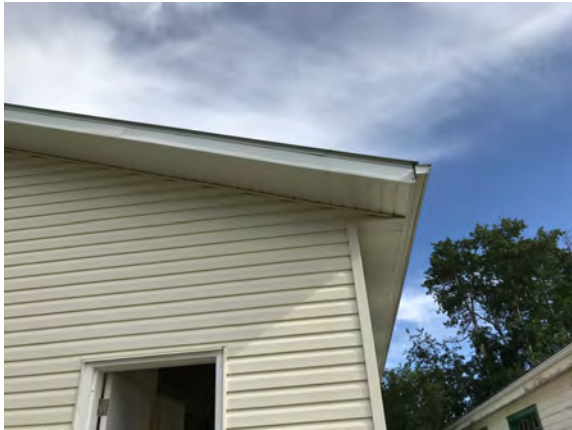
North Peace Fair Grounds - Washroom Building - B201008
