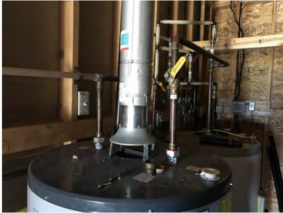
North Peace Fair Grounds - Washroom Building - D202001
