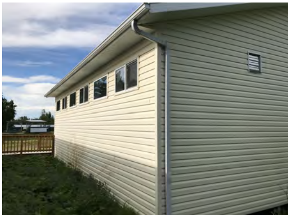
North Peace Fair Grounds - Washroom Building - B202001
