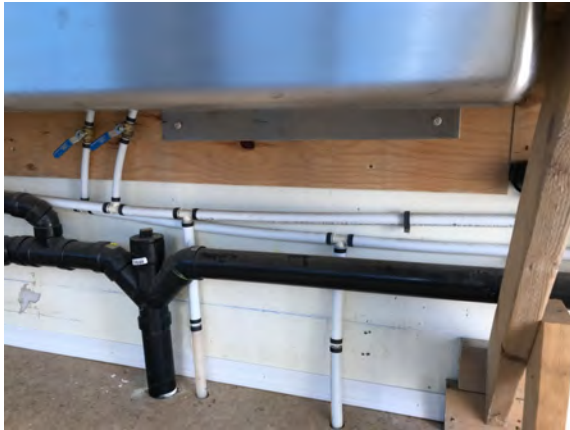
North Peace Fair Grounds - Washroom Building - D203001
