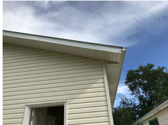
North Peace Fair Grounds - Washroom Building - B201025
