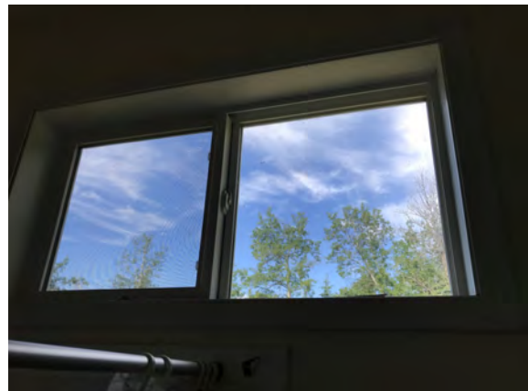
North Peace Fair Grounds - Washroom Building - B202001
