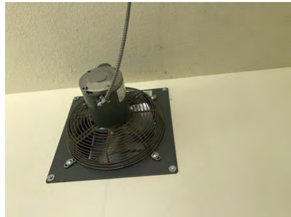
North Peace Fair Grounds - Washroom Building - D304031
