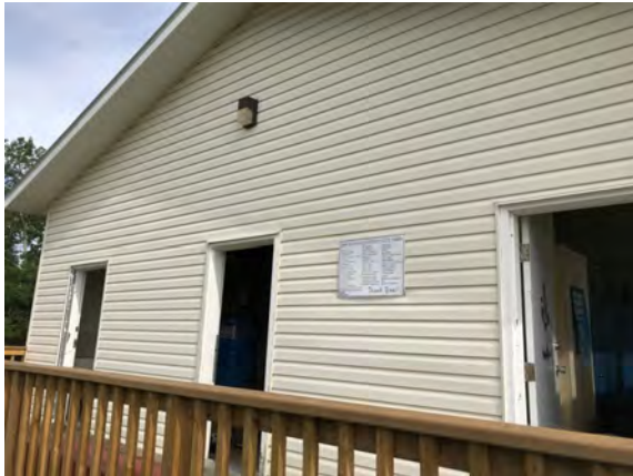
North Peace Fair Grounds - Washroom Building - D502041
