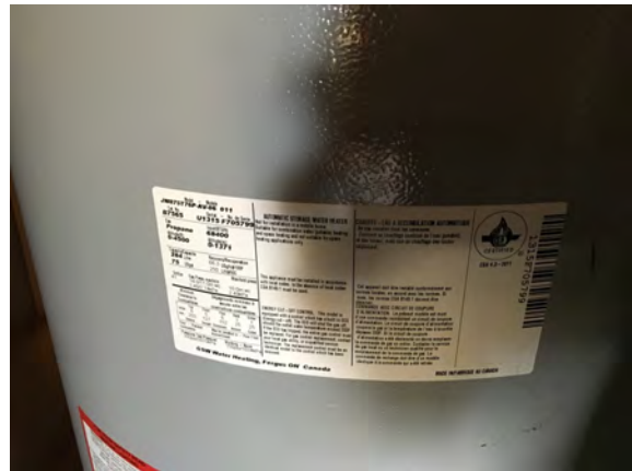
North Peace Fair Grounds - Washroom Building - D202033
