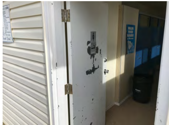
North Peace Fair Grounds - Washroom Building - B203024
