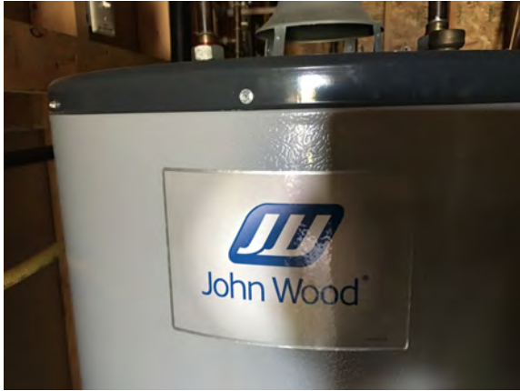
North Peace Fair Grounds - Washroom Building - D202033
