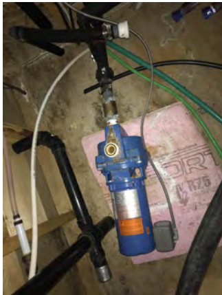
North Peace Fair Grounds - Washroom Building - D202006
