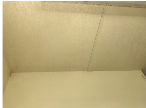
North Peace Fair Grounds - Washroom Building - C303006
