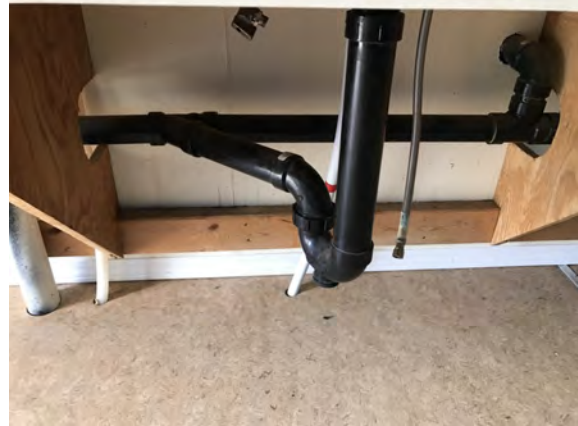
North Peace Fair Grounds - Washroom Building - D203001
