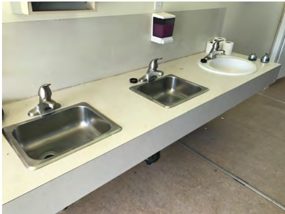
North Peace Fair Grounds - Washroom Building - D201003
