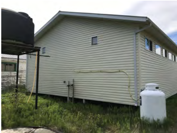
North Peace Fair Grounds - Washroom Building - B301005
