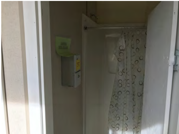
North Peace Fair Grounds - Washroom Building - C102022
