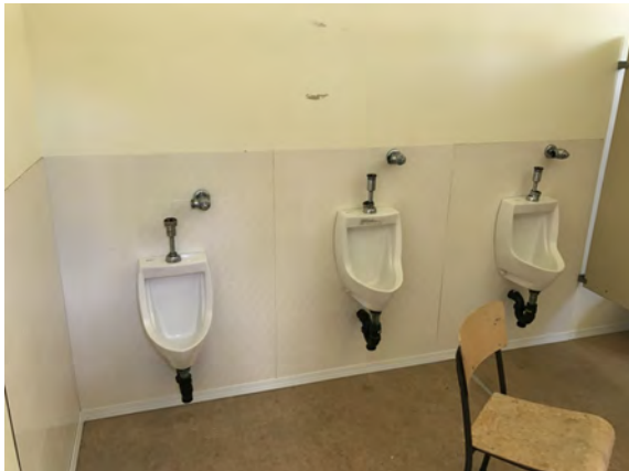
North Peace Fair Grounds - Washroom Building - D201002
