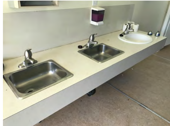
North Peace Fair Grounds - Washroom Building - C103010
