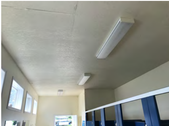
North Peace Fair Grounds - Washroom Building - D502002
