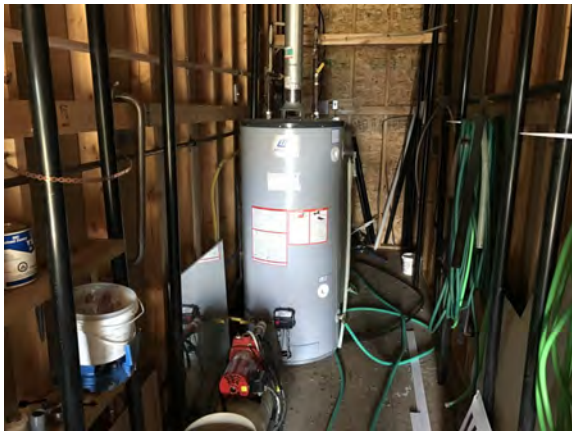
North Peace Fair Grounds - Washroom Building - D202033
