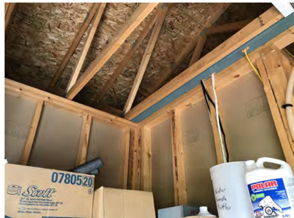
North Peace Fair Grounds - Washroom Building - B103001
