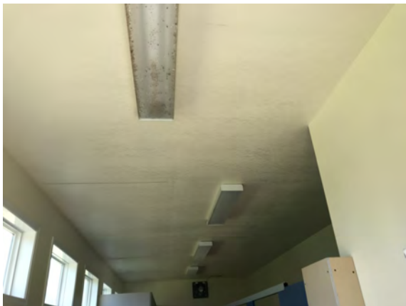
North Peace Fair Grounds - Washroom Building - C303006
