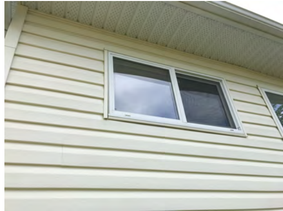
North Peace Fair Grounds - Washroom Building - B201008
