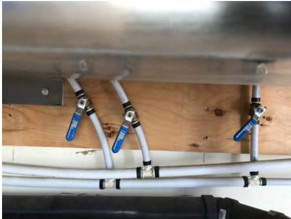
North Peace Fair Grounds - Washroom Building - D202001
