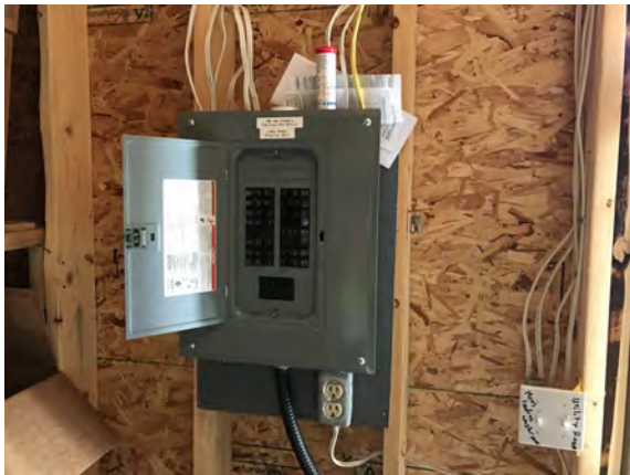
North Peace Fair Grounds - Washroom Building - D501033
