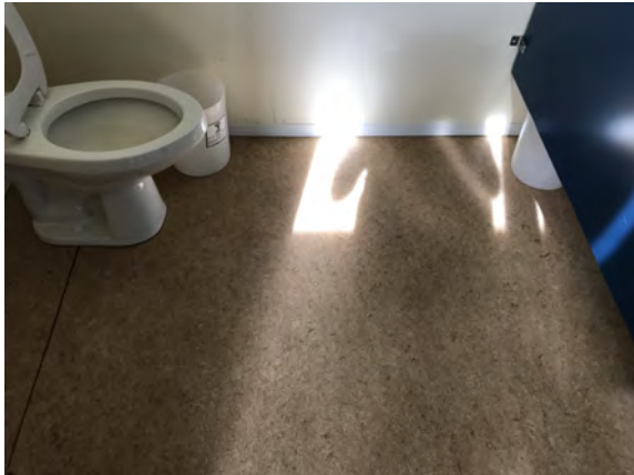
North Peace Fair Grounds - Washroom Building - C302023
