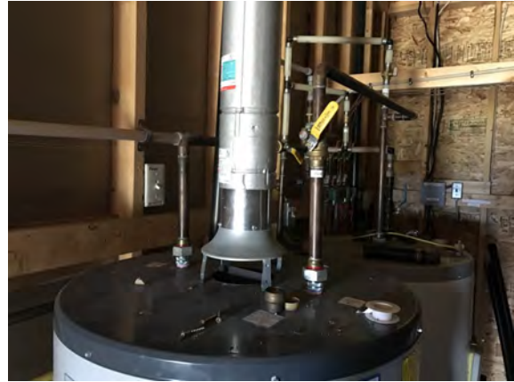
North Peace Fair Grounds - Washroom Building - D202033
