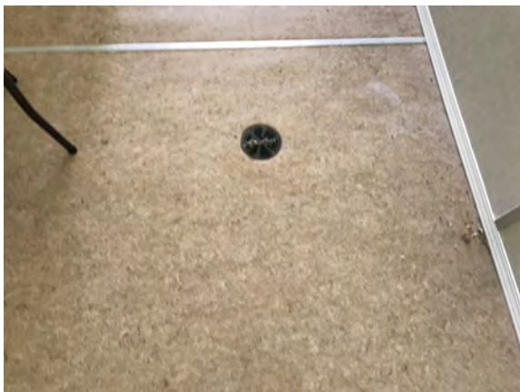
North Peace Fair Grounds - Washroom Building - C302023
