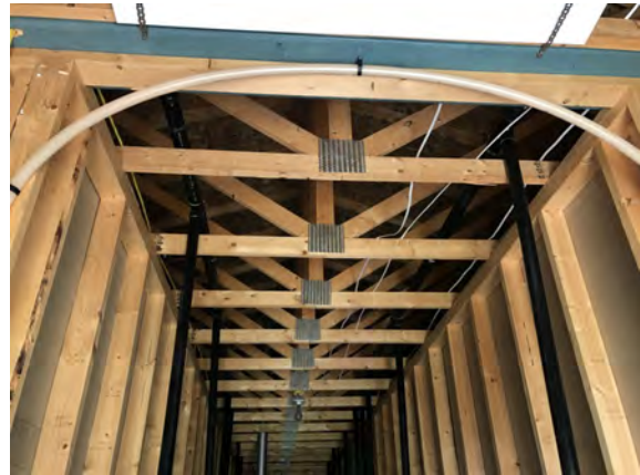
North Peace Fair Grounds - Washroom Building - B103001
