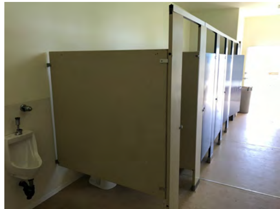
North Peace Fair Grounds - Washroom Building - C103026
