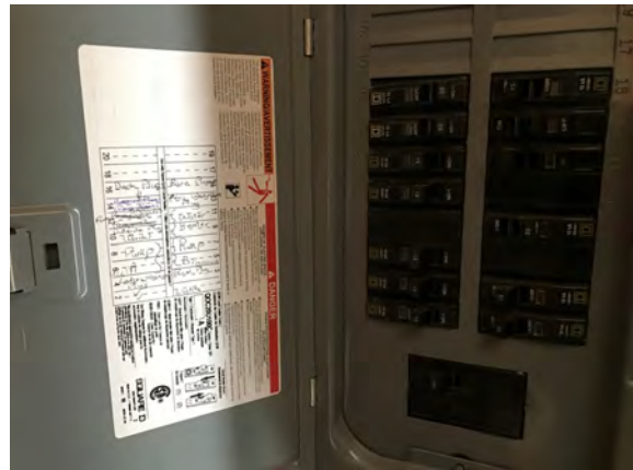
North Peace Fair Grounds - Washroom Building - D501033
