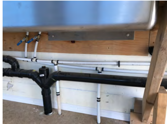
North Peace Fair Grounds - Washroom Building - D202001
