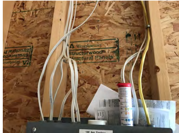
North Peace Fair Grounds - Washroom Building - D502001
