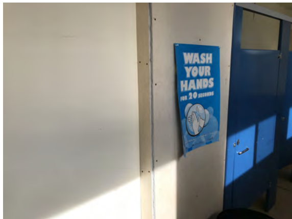
North Peace Fair Grounds - Washroom Building - C101001
