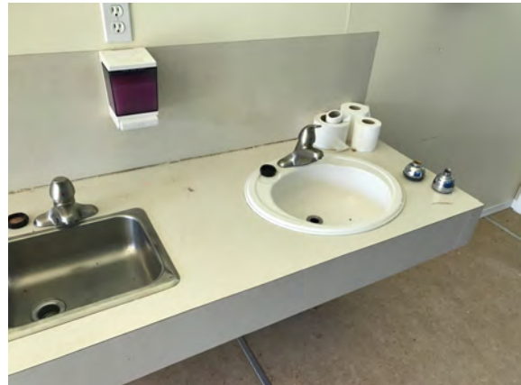
North Peace Fair Grounds - Washroom Building - D201003
