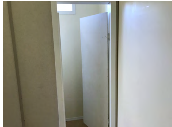
North Peace Fair Grounds - Washroom Building - C102022
