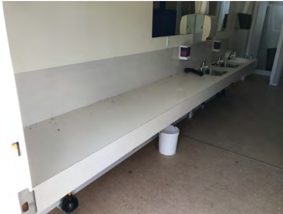
North Peace Fair Grounds - Washroom Building - C103010
