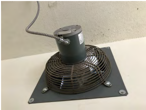
North Peace Fair Grounds - Washroom Building - D304031
