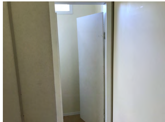
North Peace Fair Grounds - Washroom Building - C101001
