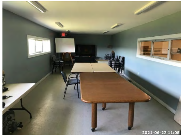
Newer LED lighting in the Apparatus Room
