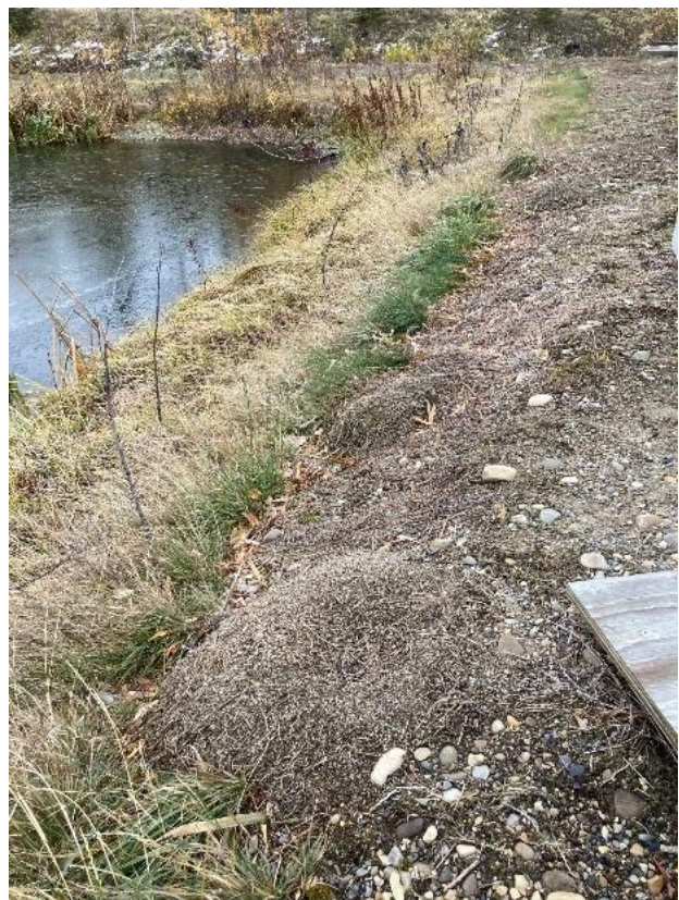
Figure 2: Muskrats Burrows between cell 4 & 5
