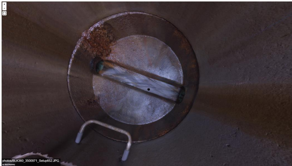
Figure 6: Infiltration Stains and Minor Encrustation Near Base Joint of SMH-02
