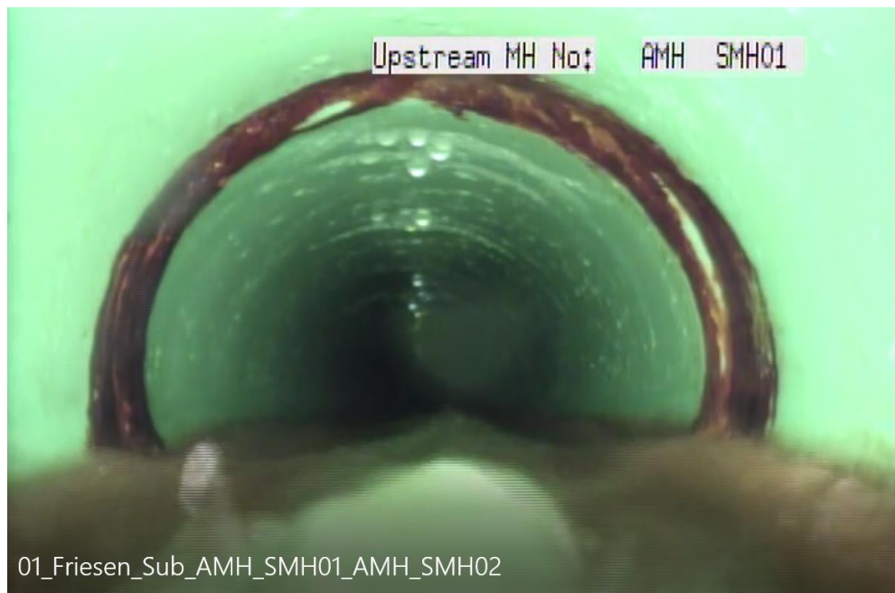
Figure 3: Circumferential Crack with Minor Infiltration
