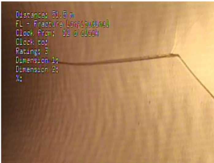
Figure 9 - Longitudinal Fracture in Overflow Pipe
