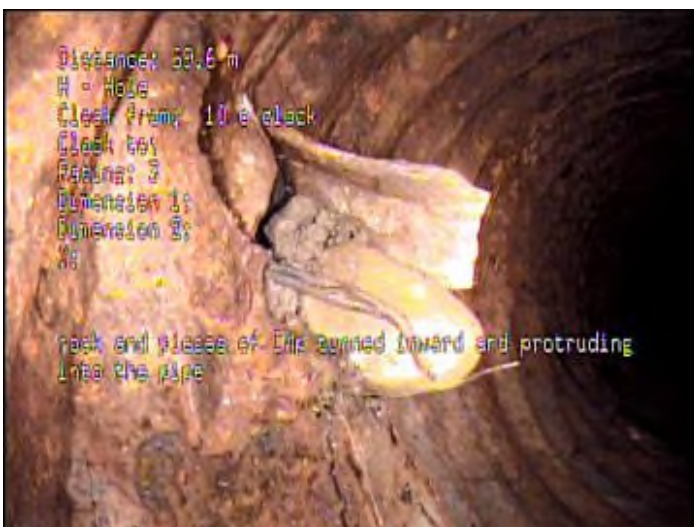
Figure 11 - Protrusion in Steel Outfall Pipe
