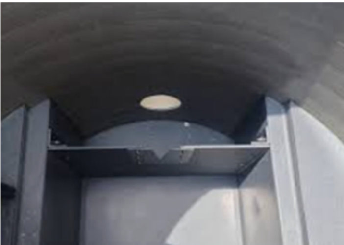
Figure 14 - Example of V-Notch Weir
