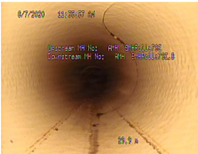
Figure 10 - Spiral Fracture in Overflow Pipe
