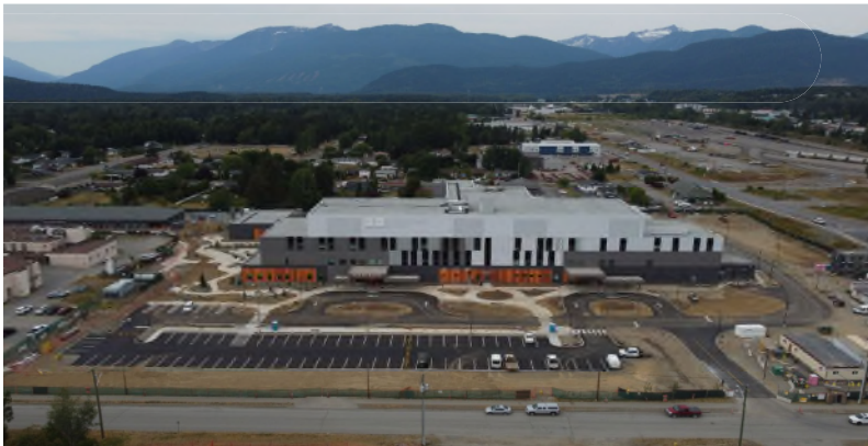
Landscaping & Civil (East Side)
