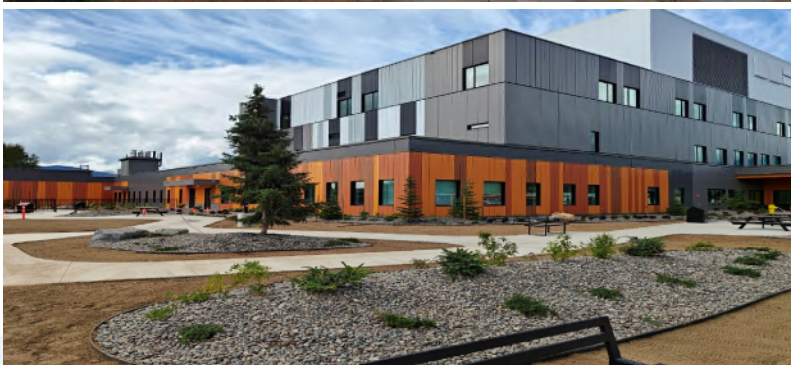
Landscaping & Civil (East Side)
