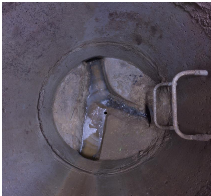
Figure 13: Standing Water in Channels of SMH-01F (Final Manhole before Harper Lift Station).
