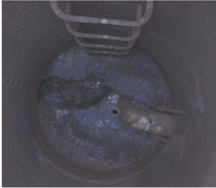
Figure 15: Drop Structure in Good Condition Based on Visual Inspection, with Restraints Intact. Rusting is present on the restraint hardware, but bolt threading and nut shape remain distinct and visible.
