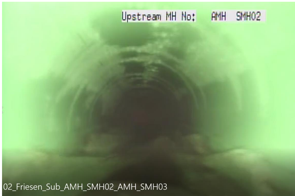
Figure 4: CCTV Image Taken During Period of Moderate Flow Flow may have led to a hydraulic jump condition causing an instance of underwater camera
