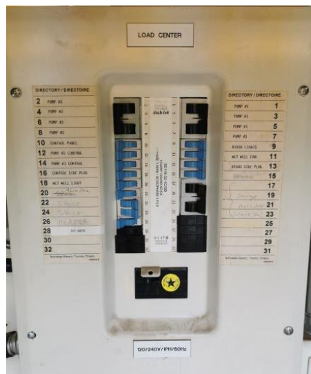
Figure 12: Electrical Panel with Federal Pioneer Breakers
