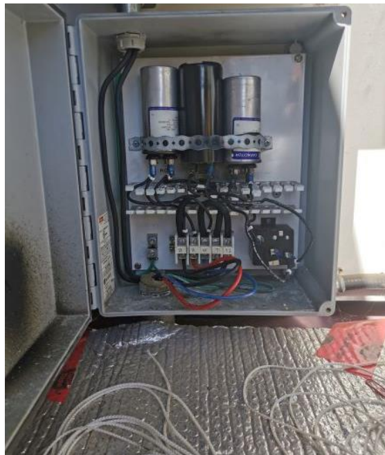
Figure 14: Capacitor Cabinet with Burn Mark
