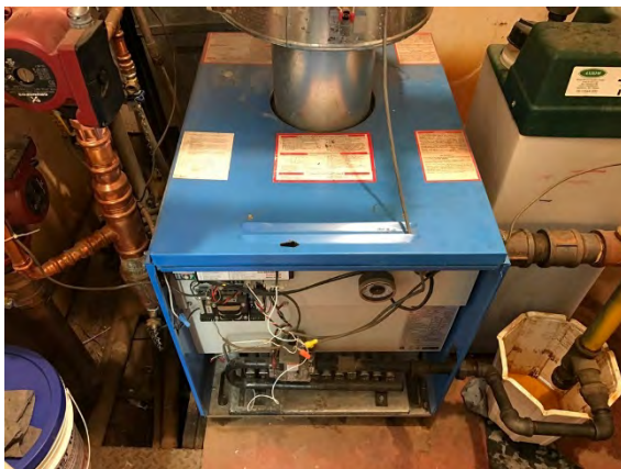
Main heating boiler
