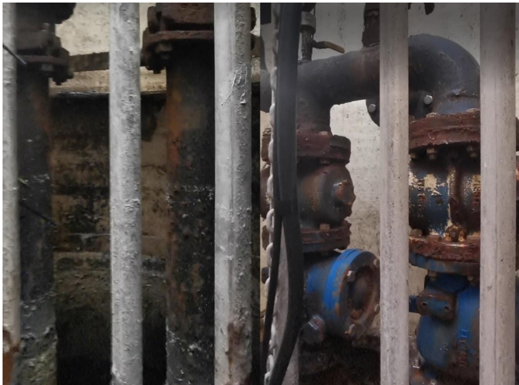
Figure 4: Rusted Pipes, Flanges, and Valves in the Wet Well
