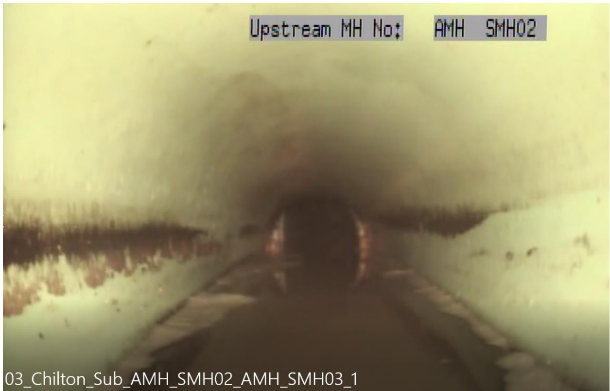
Figure 16: Sags in Pipe Grade Causing Standing Water between SMH-02 and SMH-03
