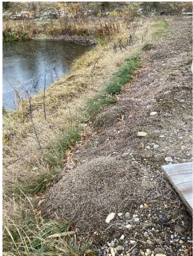
Figure 2: Muskrats Burrows between cell 4 & 5
