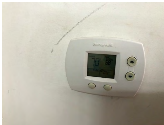
Non-Programmable thermostat for control of the heating
