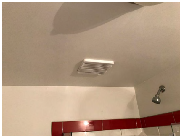
View of ceiling mounted bathroom exhaust fan
