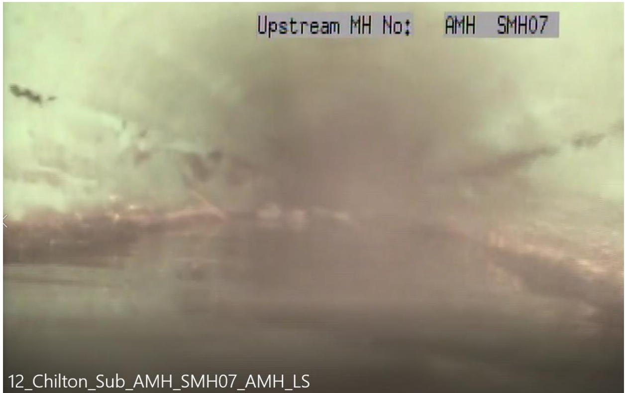
Figure 19: Debris Blocking Sewer Main Leading to Chilton Lift Station
