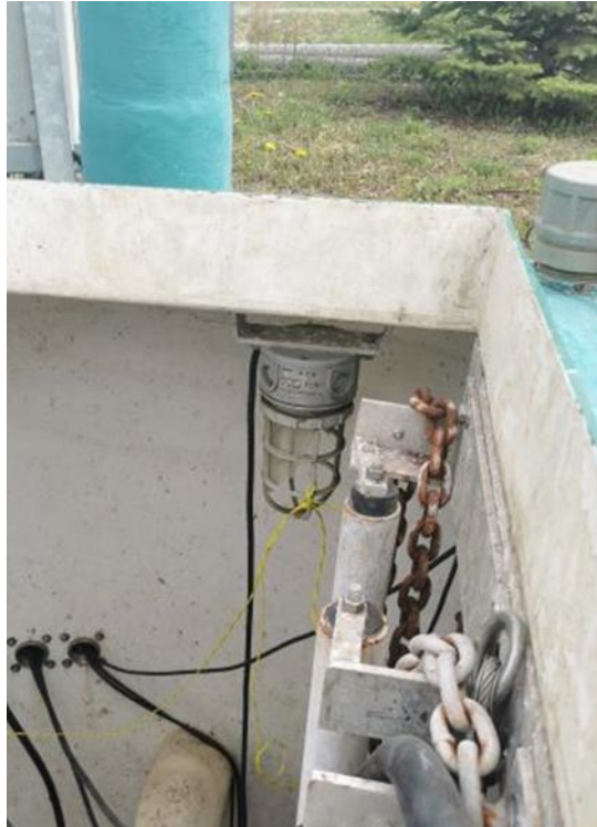
Figure 9: Damaged Explosion Proof Fixture (Light Bulb)
