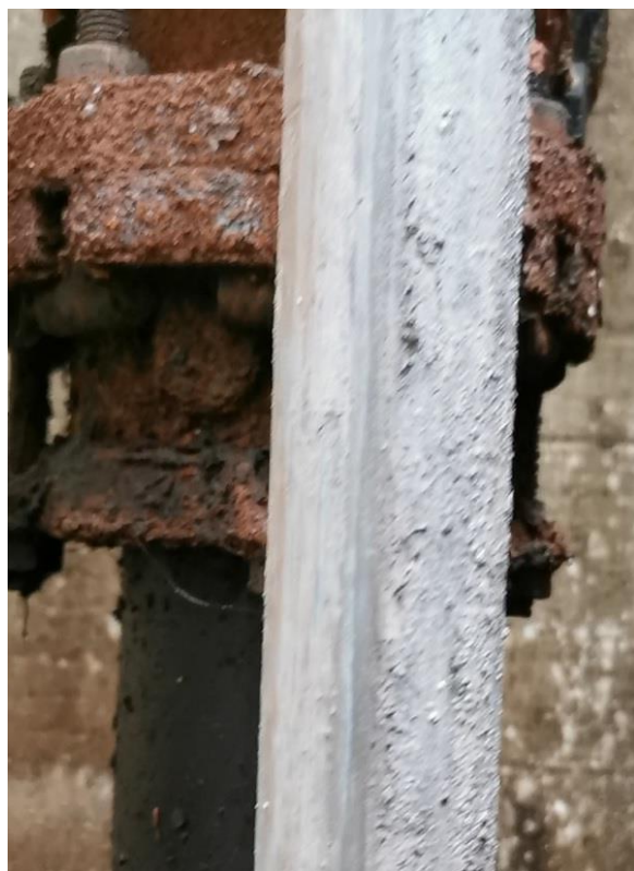
Figure 4: Rusted Pipe and Flange in the Wet Well
