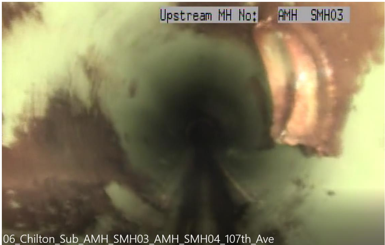
Figure 17: Intruding Service Caused CCTV Inspection to be Abandoned; Service Installed Correctly and Not Defective
