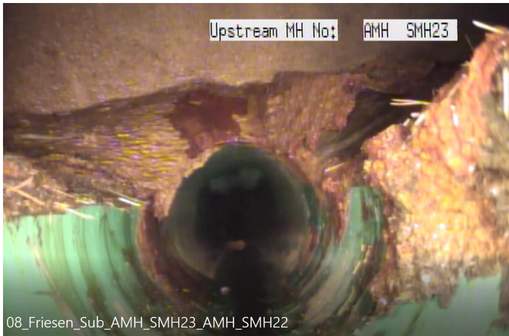
Figure 7: Encrustation Around Benching of SMH-22
