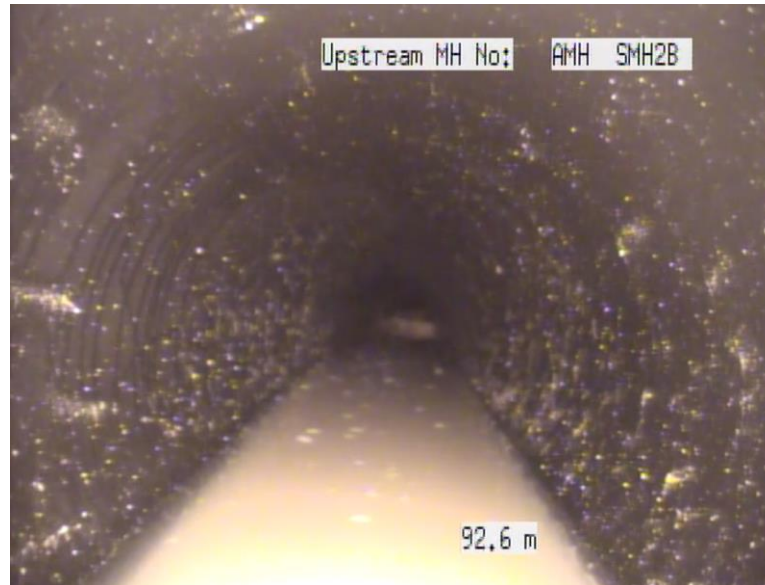
Figure 12: Gravel and Water Level Obstruction Caused by Pipe Sag Between SMH-02B and SMH-02C
