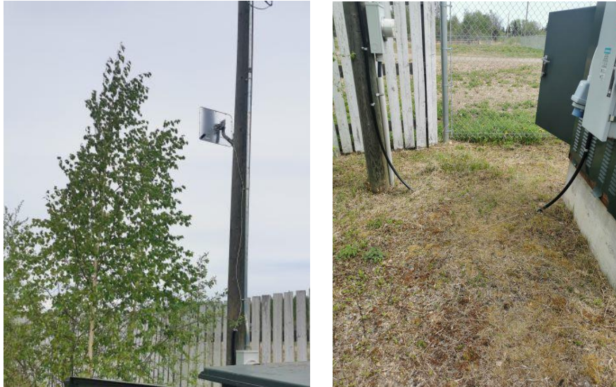
Figure 11: Antenna and Improperly Installed Cable
