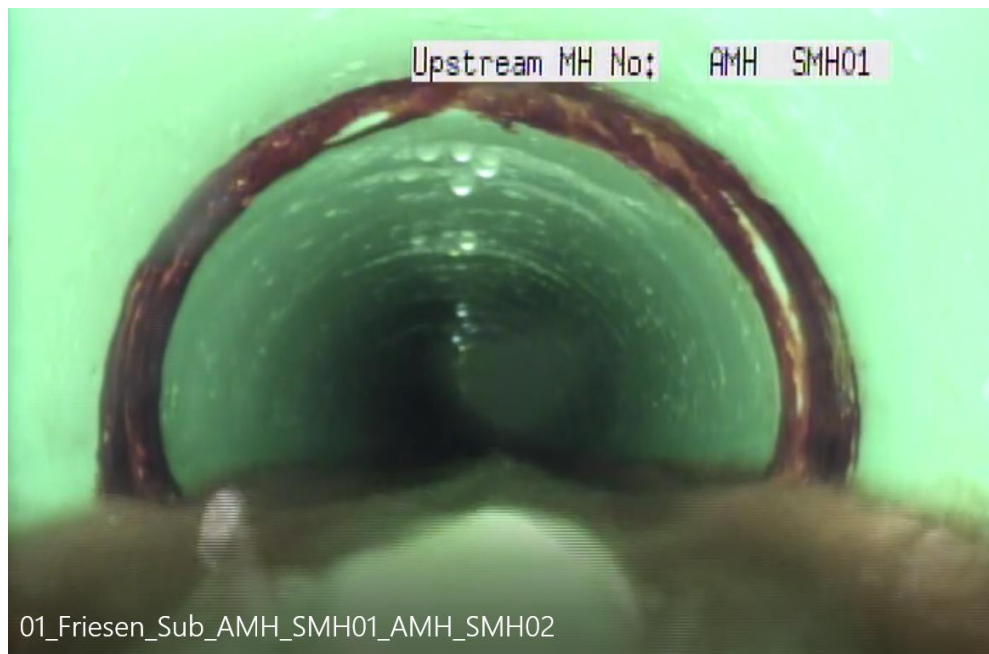
Figure 3: Circumferential Crack with Minor Infiltration
