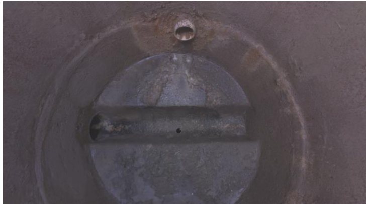
Figure 14: Break in Service Connection to SMH-02B. This service does not have a drop structure or benching to direct flows.
