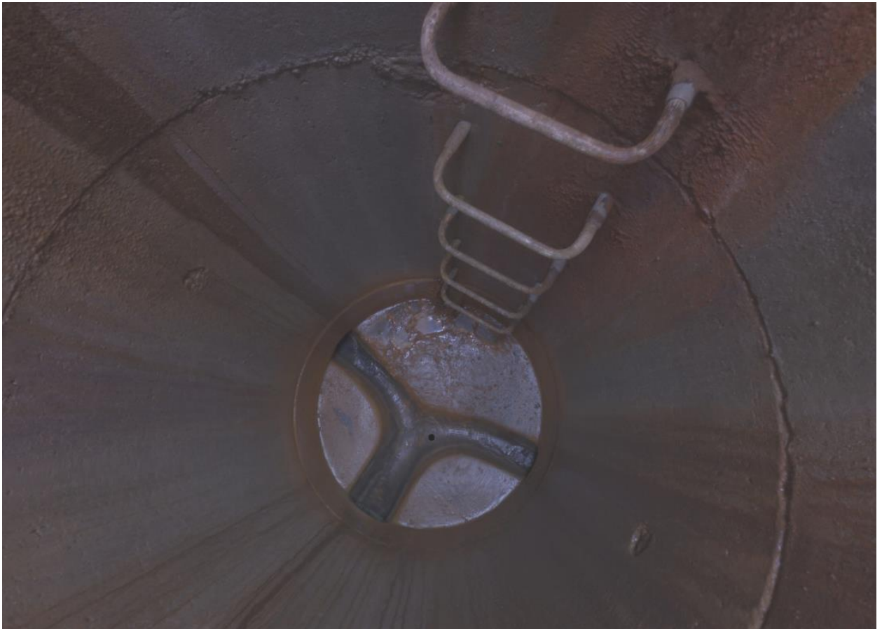
Figure 20: Some Minor Infiltration Staining and Encrustation in SMH-01
